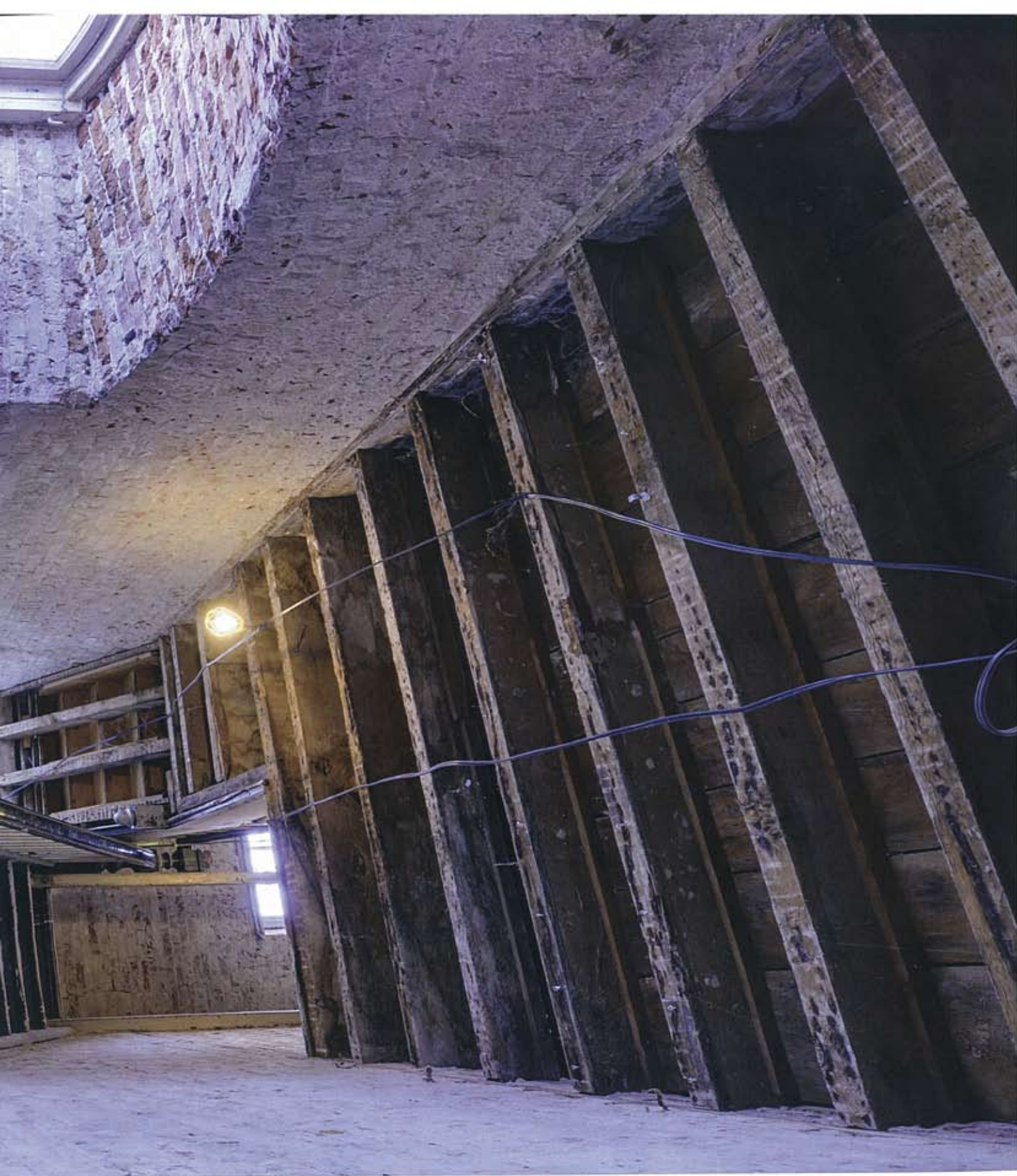
Stairwell in former Governor's residence quarters
